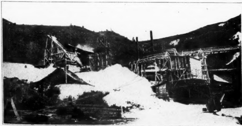
A General View of the Calcining Plant.
